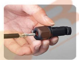
Put the crimped male pin into male housing tightly until it's set by "Click".
